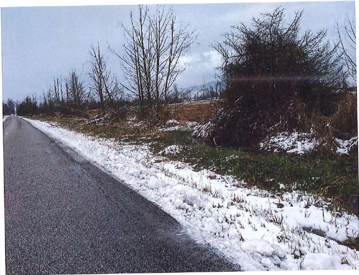
Photo 2: View of the ditch on the southside of Kneuman Rd looking east. Water is slow moving with a fair amount of vegetation. There is a fallen tree, potentially causing a blockage and slower moving flow in the ditch.
