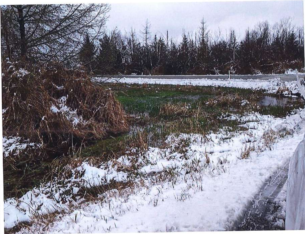
Photo 1: A view of the roadside ditch at the corner of Barbo Rd and Kneuman Rd. The current ditch conditions show a backed-up channel slow moving water with a fair amount of vegetation.
