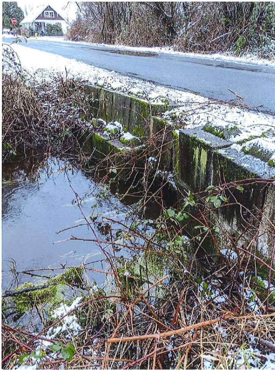
Photo 8: There are large culverts in the creek downstream of the project site. They were estimated visually to be roughly 4-ft in diameter. Conditions made it difficult to access the culverts safely for an accurate measurement.
