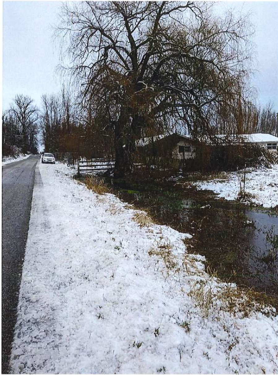
Photo 3: The ditch appears to bottleneck as it approaches the culvert crossing. Ditch continues to have a fair amount of vegetation.
