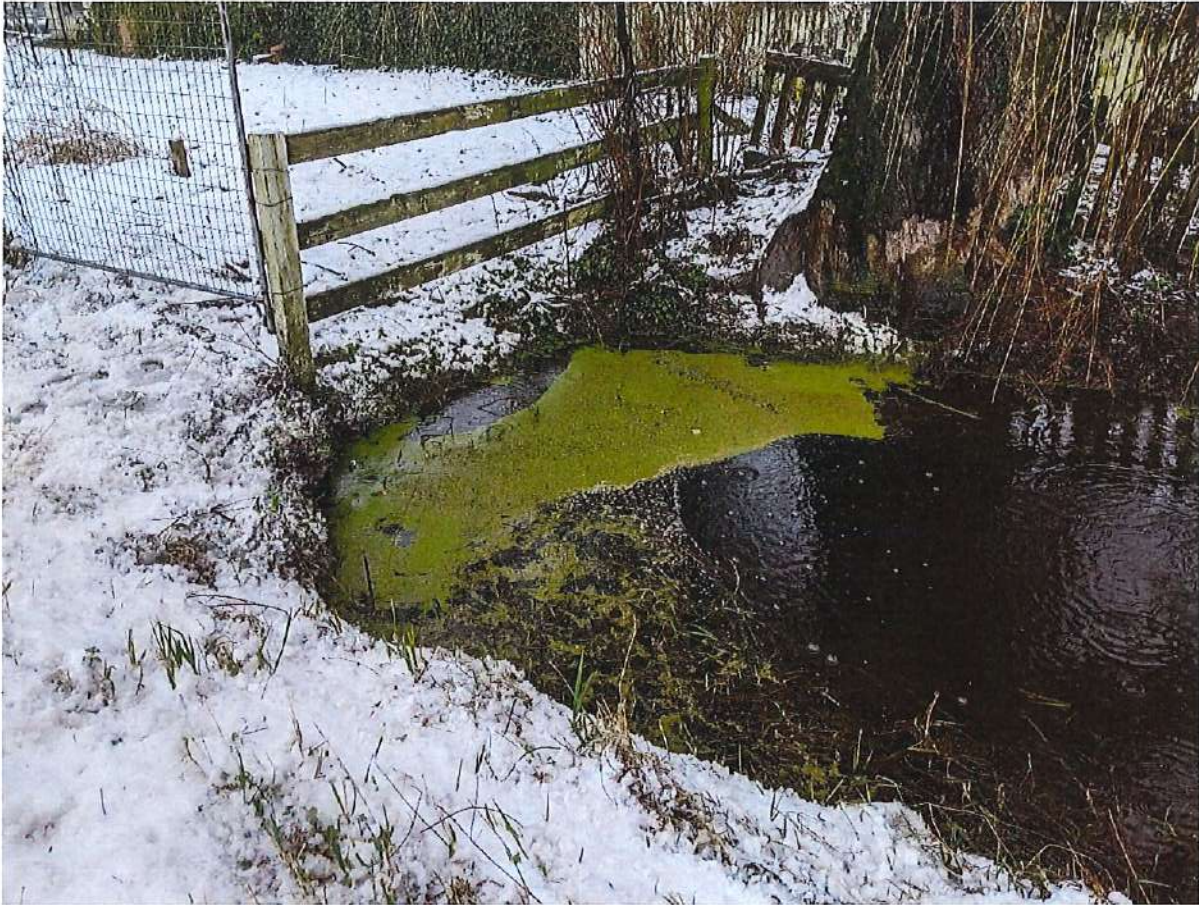
Photo 4: Upstream of the culvert inlet. Flow depth is roughly 5.5-ft to 6.5-ft and the top width is roughly 13-ft to 15-ft in this area. Culvert is fully submerged and could not be surveyed at this time.
