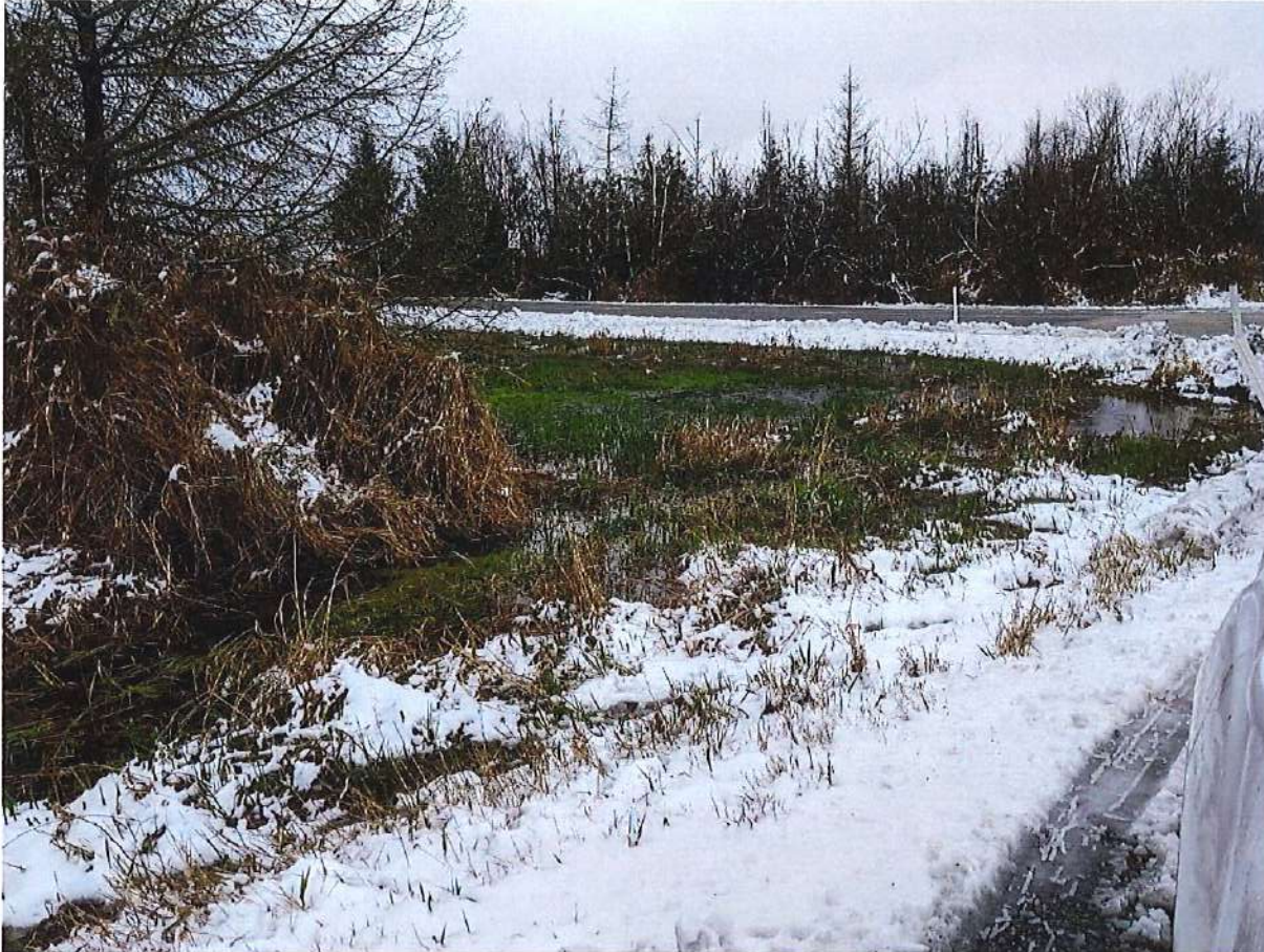
Photo 1: A view of the roadside ditch at the corner of Barbo Rd and Kneuman Rd. The current ditch conditions show a backed-up channel slow moving water with a fair amount of vegetation.
