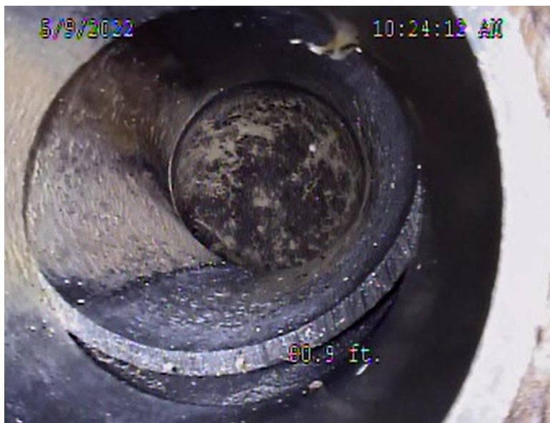
SITE 10: Separation of PCV Sewer Pipe (3 inch) under Sumas Ave. 80 feet east of Sumas Ave SSMH-4A.
