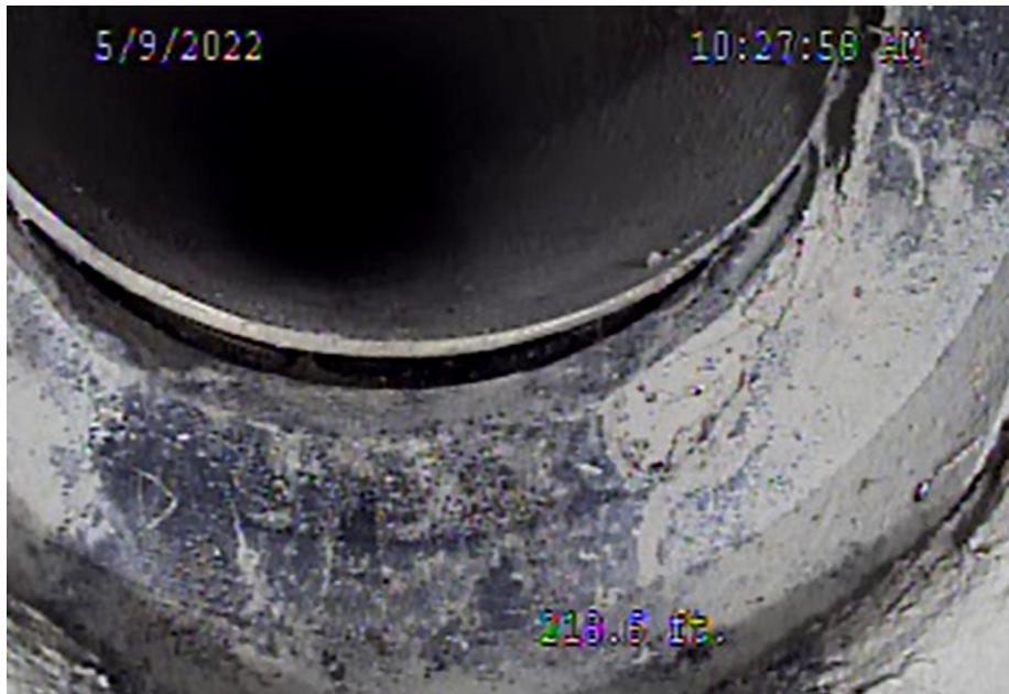
SITE 9: Separation of pipe connection between main Asbestos Concrete Sewer Pipe (8 inch) and PVC house connection pipe (3 inch) under a side street. 218 feet east of Sumas Ave SSMH-4A.
