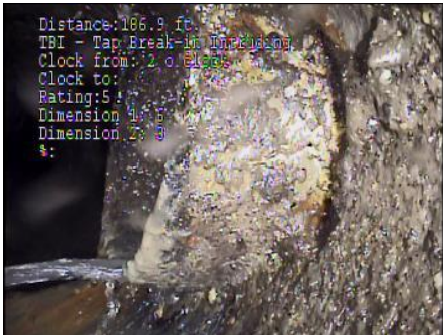
SITE 13: Side asbestos concrete (3 inch) side connection pipe shoved into main asbestos concrete Sewer Pipe (8 inch). 186 feet east of Garfield SSMH-2 under Garfield St.
