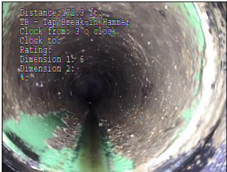
SITE 25: Separation of pipe connection between main Asbestos Concrete Sewer Pipe (8 inch) and PVC house connection pipe (3 inch) under First Street. Separation is 172 feet east of First Street SSMH-1.
