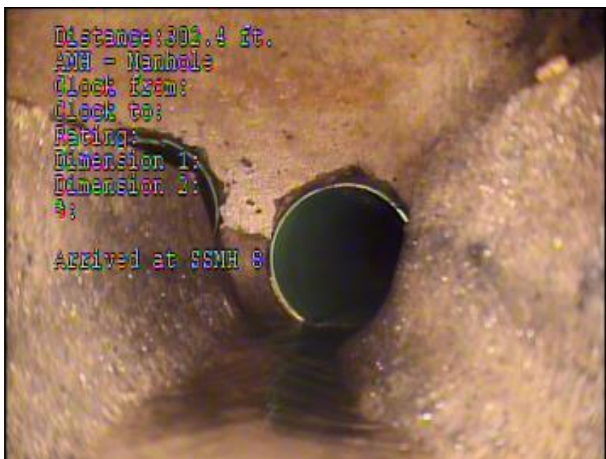
SITE 18: Damage to SSMH-8, where the manhole trough has been misaligned from the pipe connection.
