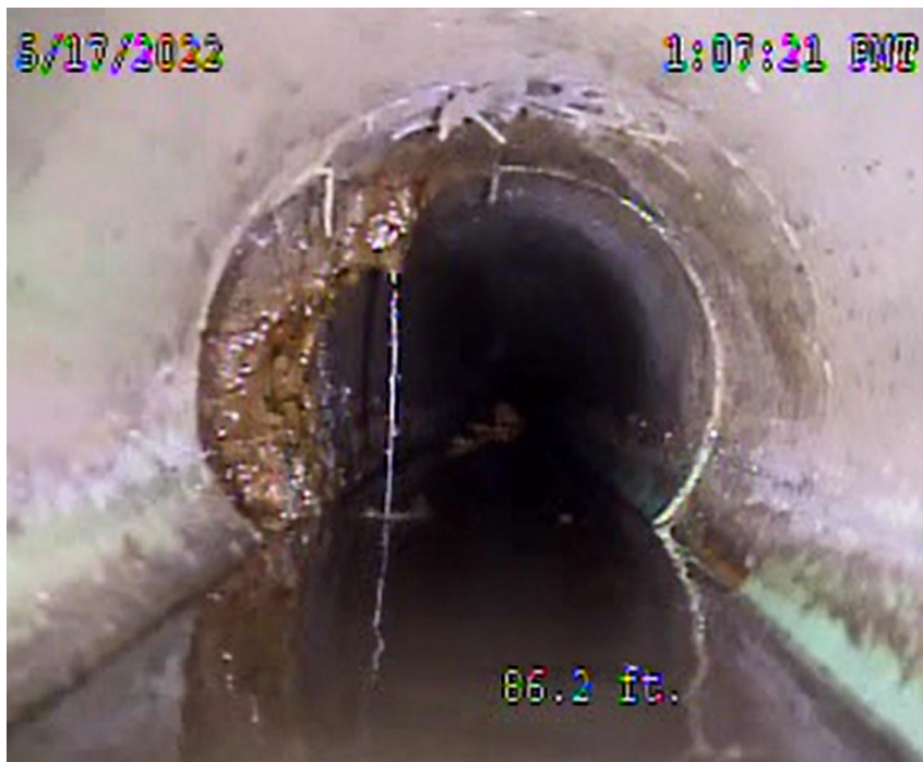
SITE 26: Leaking pipe joint on main PVC sewer pipe (8 inch). 88 feet west of Second St SSMH-7.
