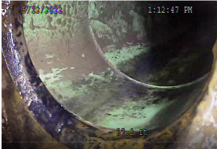
SITE 3: Separation of PVC pipe (3 inch) from main Asbestos Cement Sewer Pipe (8 inch) connection between Lawson St. SSMH-2B and Lawson St. SSMH-2. Crack is 39 feet west of Lawson St. SSMH-2B.
