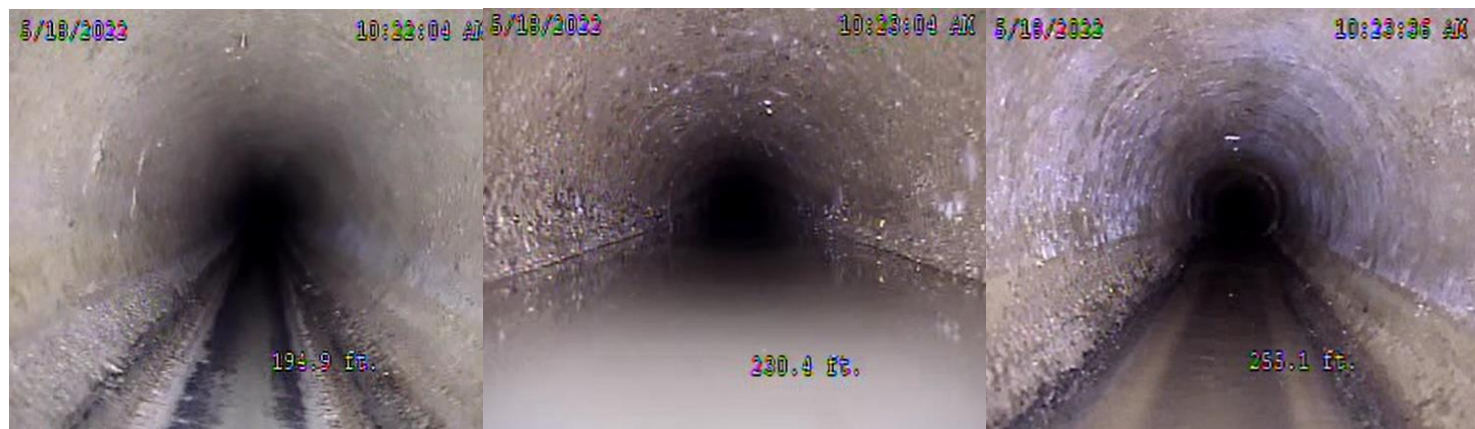
SITE 24: Deep ~ 3-inch deflection in 8-inch Asbestos Concrete Sewer Pipe between Cleveland SSMH-5 and Lawson SSMH-4. Deflection is approximately 60 feet long and located 194 feet north of Cleveland SSMH-5.
