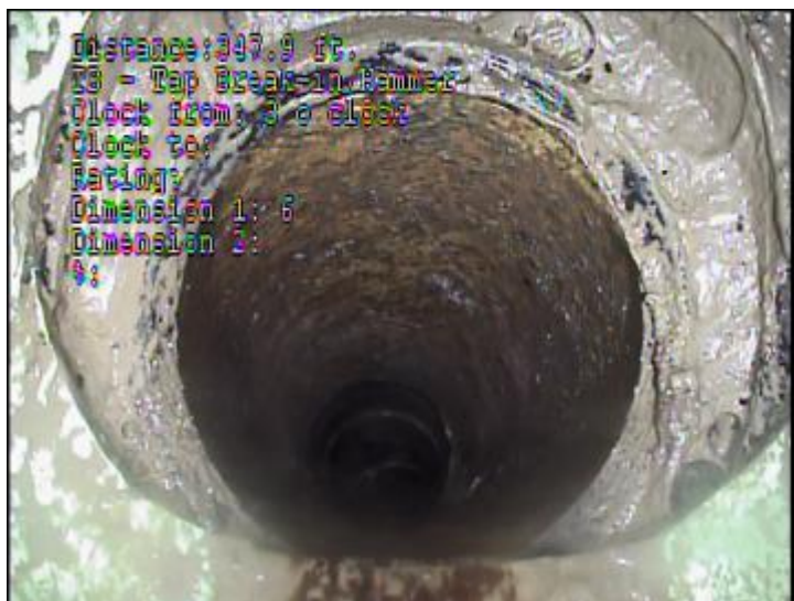
SITE 6: Separation of pipe connection between main PVC Sewer Pipe (8 inch) and PVC house connection pipe (3 inch) under Morton Street. 347 feet west of Morton St. SSMH-3A.
