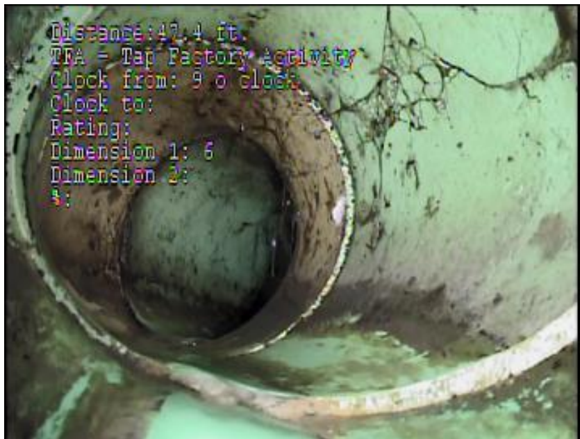
SITE 4: Crack in Noble St. PVC pipe (3 inch) . Crack is 47.4 feet west of Noble St. SSMH-1A.
