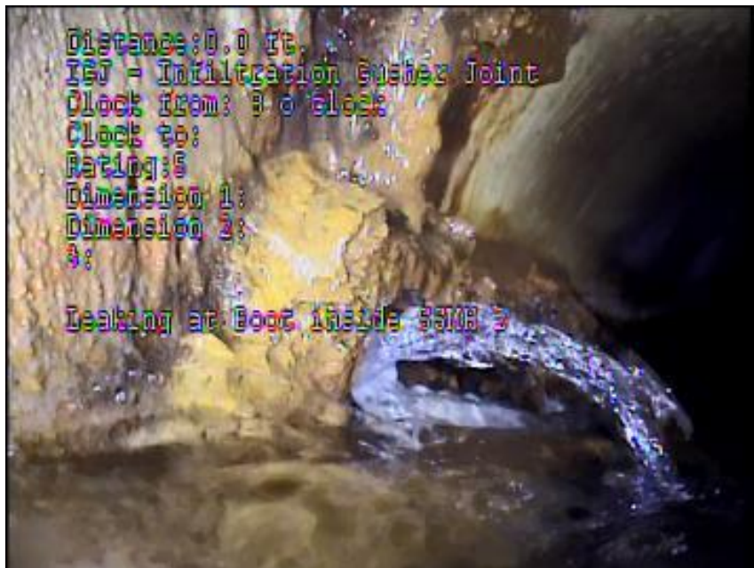
SITE 20: Leaking at joint connection between 8-inch PVC sewer main line and EPL SSMH-2.
